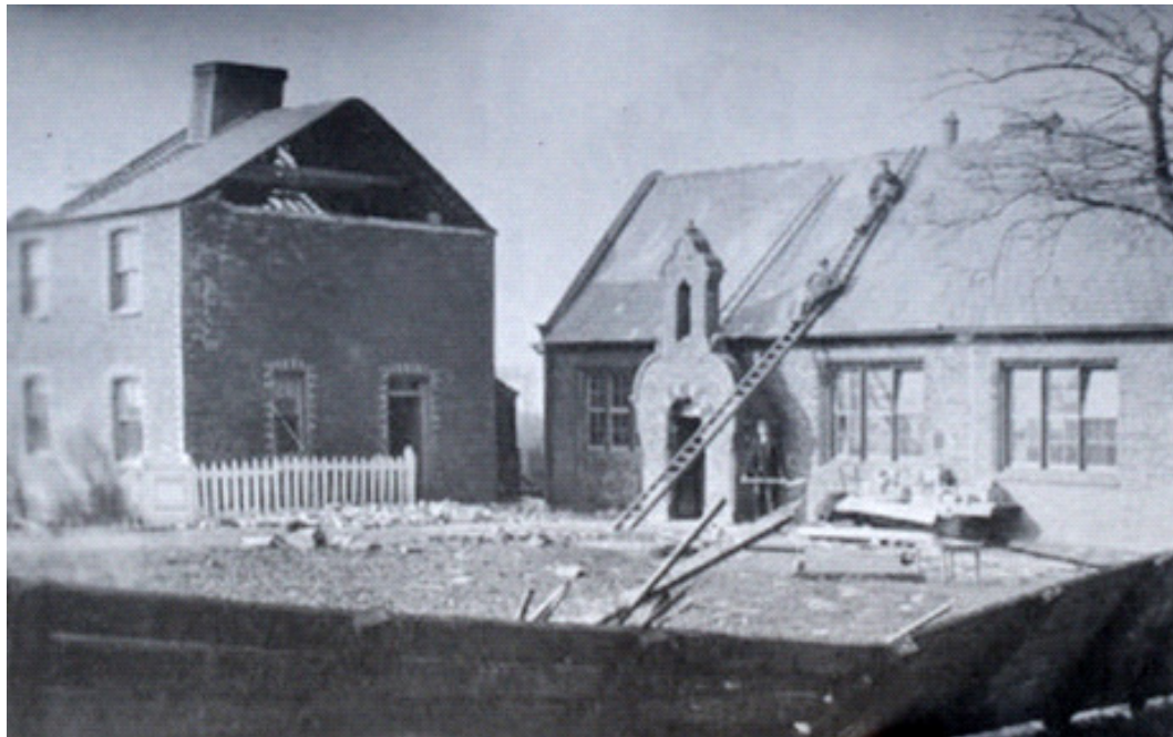
Storm damage being repaired at Saltfleetby School in 1908
