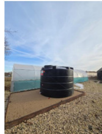
The new tank that feeds the irrigation system.
